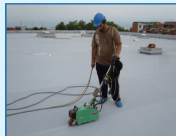
屋面PVC防水膜焊接
